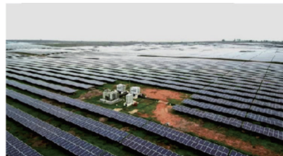
Rewa Ultra mega solar plant, Madhya Pradesh 750 MW
