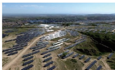
Datong Solar Power plant, China
