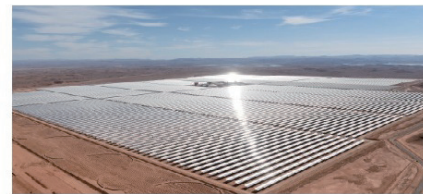
Noor Solar Park, Morocco
