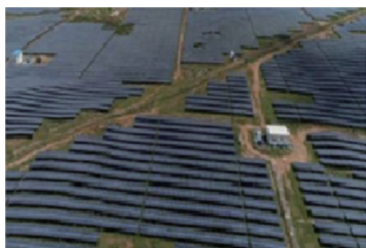
Ananthapuram ultra mega solar park, Andhra Pradesh 1000 MW
